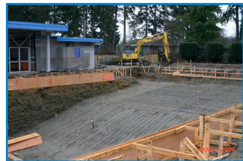
Pool w/Rebar for Concrete
