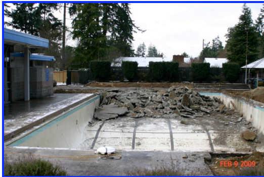
Pool after Day 1 Construction
